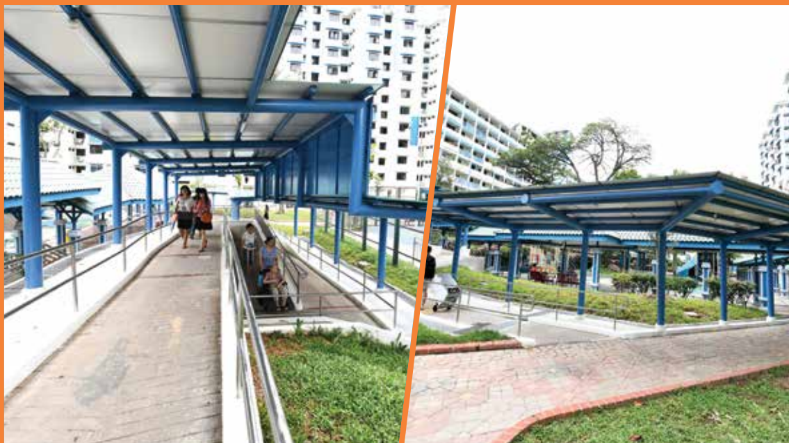
Construction of shelter over existing ramp at Blk 108 Lor 1 Toa Payoh to Blk 205 Toa Payoh North
